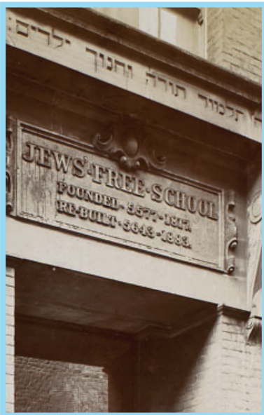
The entrance to the Bell Lane site
